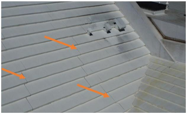
**Roof Surface Areas** - Visual elevations of surface areas identified to be in good overall condition with slight separation/cracking that should be monitored for any further separation. Concrete roof separation/cracking does not always mean a leak will occur, but a solid roof area should always be maintained.
