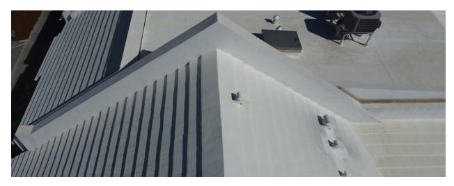
**Roof Surface Areas** - Visual elevations of surface areas identified to be in good overall condition with slight separation/cracking that should be monitored for any further separation. Concrete roof separation/cracking does not always mean a leak will occur, but a solid roof area should always be maintained.
